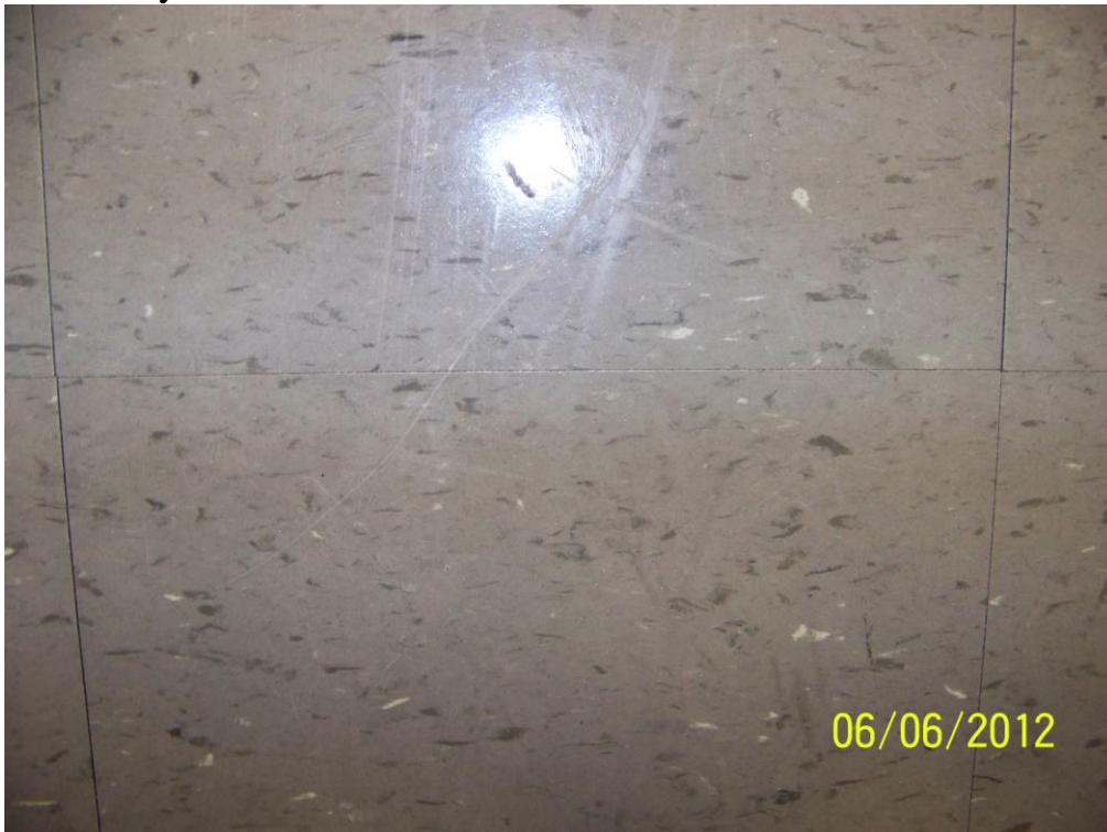
Homogeneous Material No. 30 – 12”x12” Floor Tile, Gray with Dark Gray and White Flecks
