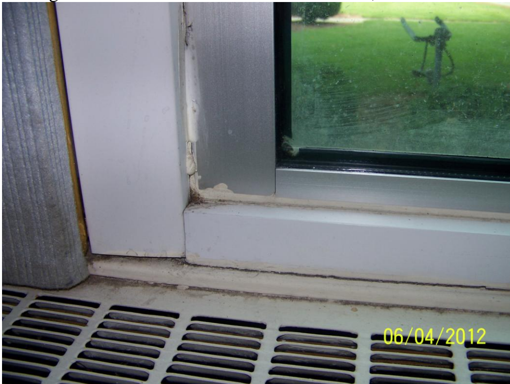
Homogeneous Material No. 14 – Window Caulk, Off-White
