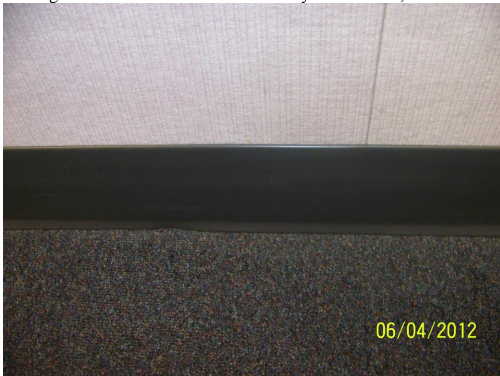
Homogeneous Material No. 21 – 6” Vinyl Cove Base, Dark Green
