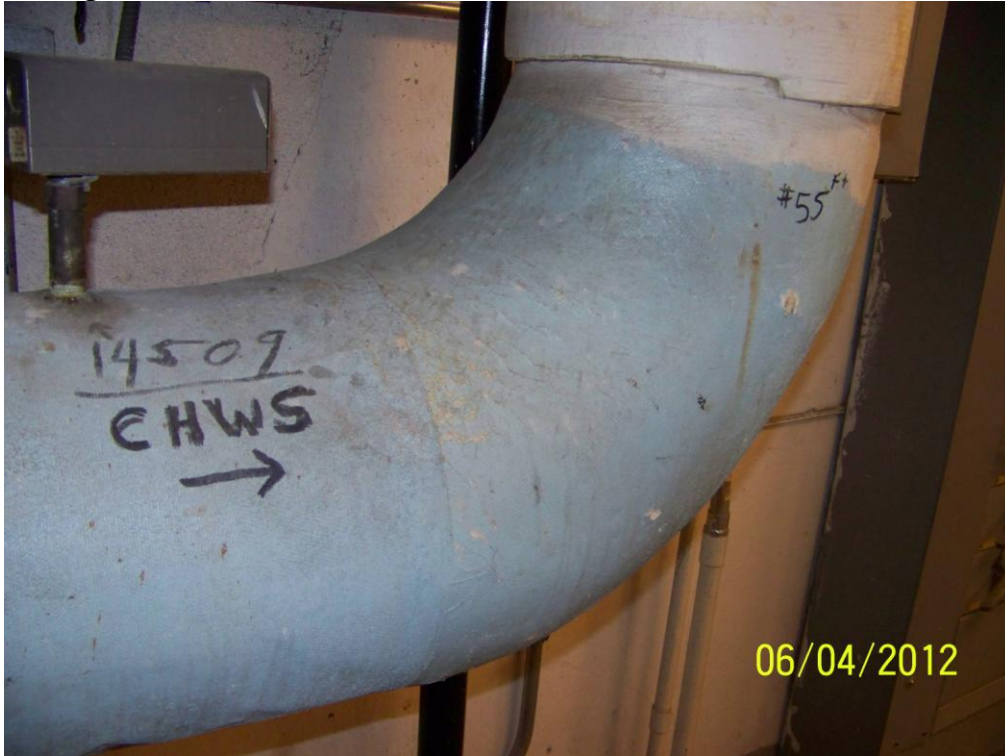
Homogeneous Material No. 1 – Mud Compound Insulation on Fiberglass Lines – Chilled Water
