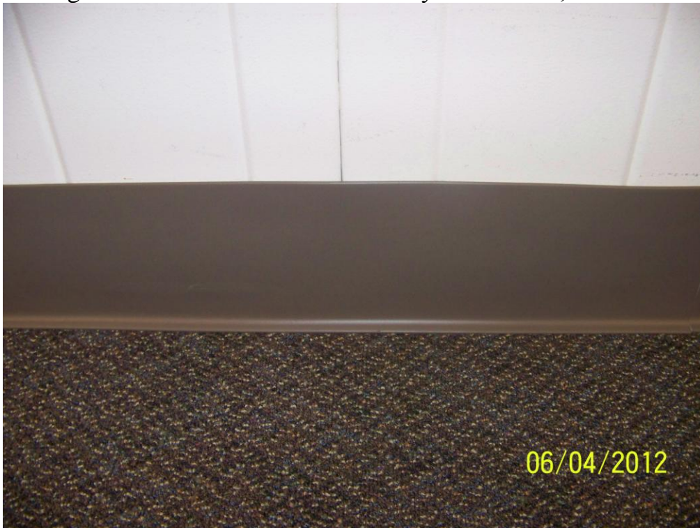
Homogeneous Material No. 16 – 6” Vinyl Cove Base, Tan
