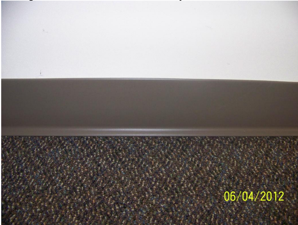
Homogeneous Material No. 13 – 4” Vinyl Cove Base, Tan
