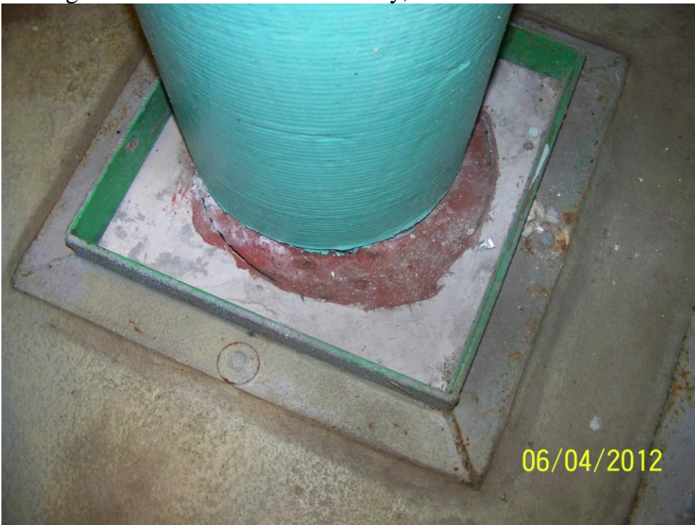
Homogeneous Material No. 10 – Putty, Red
