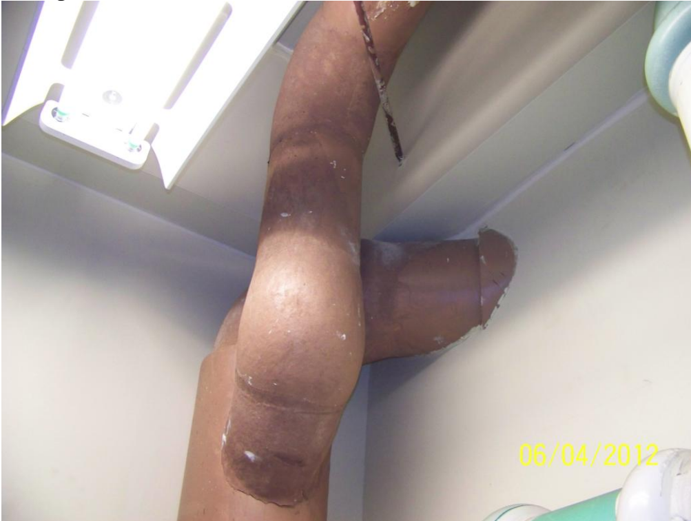
Homogeneous Material No. 9 – Mud Compound Insulation on Fiberglass Lines – Roof Drains
