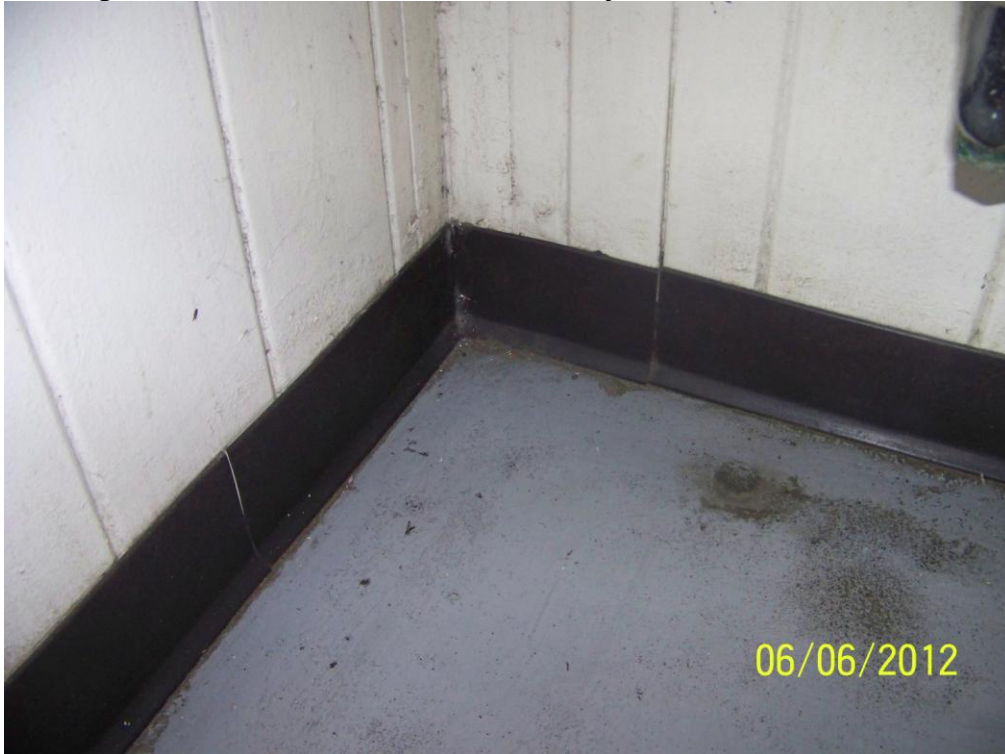
Homogeneous Material No. 33 – 4” Vinyl Cove Base, Brown
