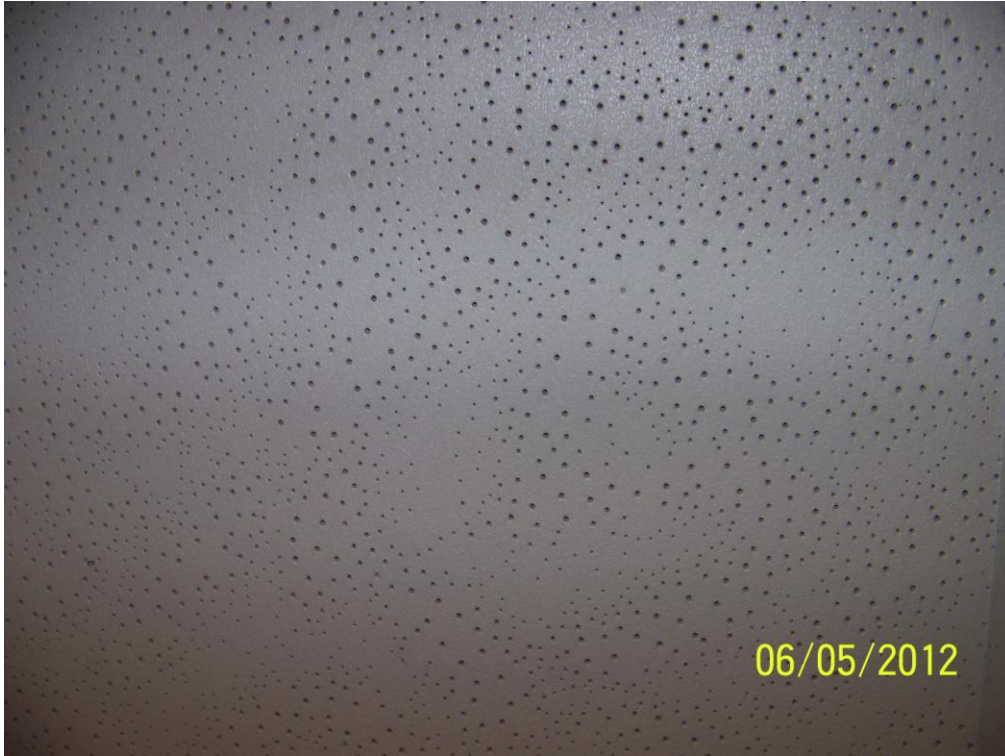
Homogeneous Material No. 29 – 2’x4’ Ceiling Tile, White, Patterned Pen Holes
