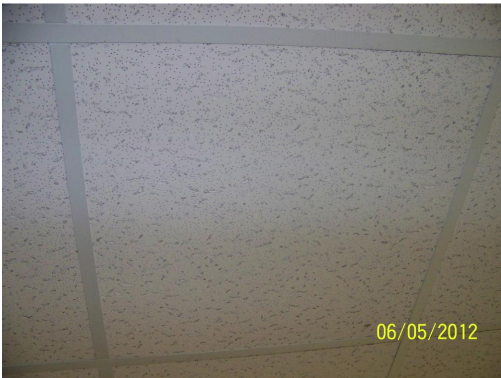
Homogeneous Material No. 26 – 2’x2’ Ceiling Tile, White, Lateral Grooves and Pin Holes
