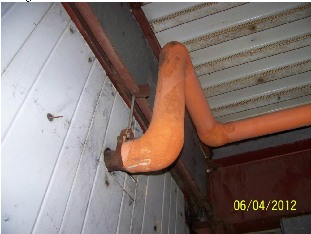
Homogeneous Material No. 6 – Mud Compound Insulation on Fiberglass Lines – Domestic Water
