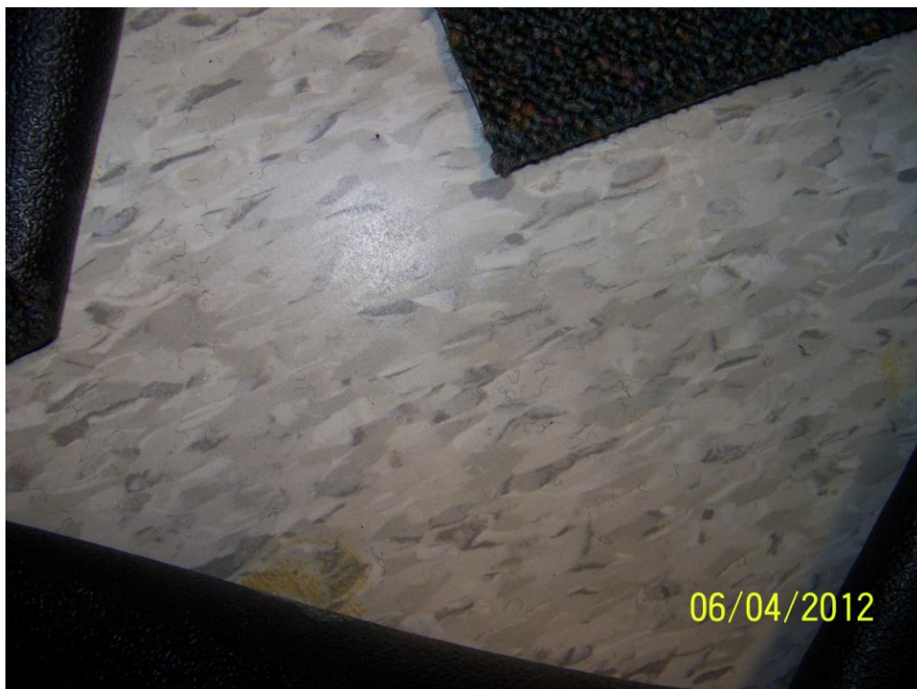
Homogeneous Material No. 22 – 9”x9” Floor Tile, Rose, White and Brown Streaks
