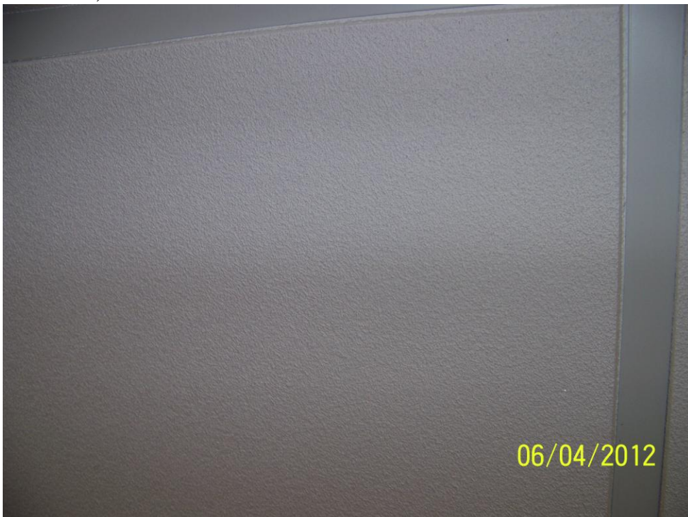
Homogeneous Material No. 20 – 2’x2’ Ceiling Tile, White, Textured, Recessed
