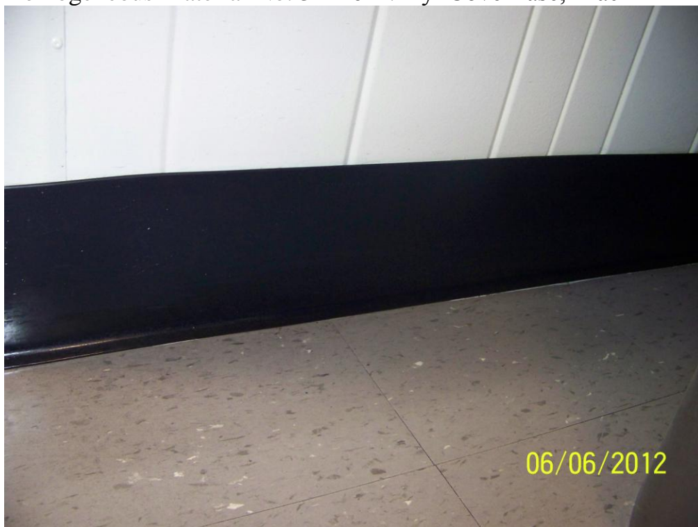
Homogeneous Material No. 31 – 6” Vinyl Cove Base, Black
