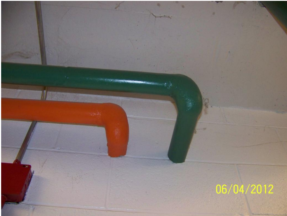
Homogeneous Material No. 3 – Mud Compound on Fiberglass Lines – Domestic Water
