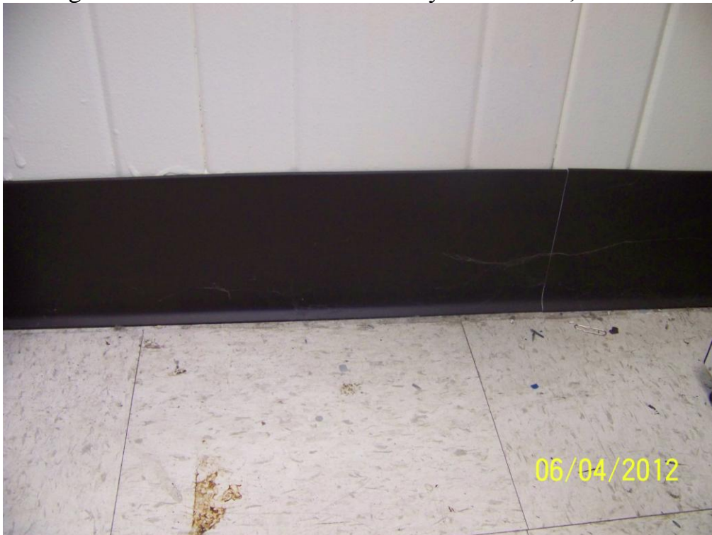
Homogeneous Material No. 18 – 6” Vinyl Cove Base, Dark Brown
