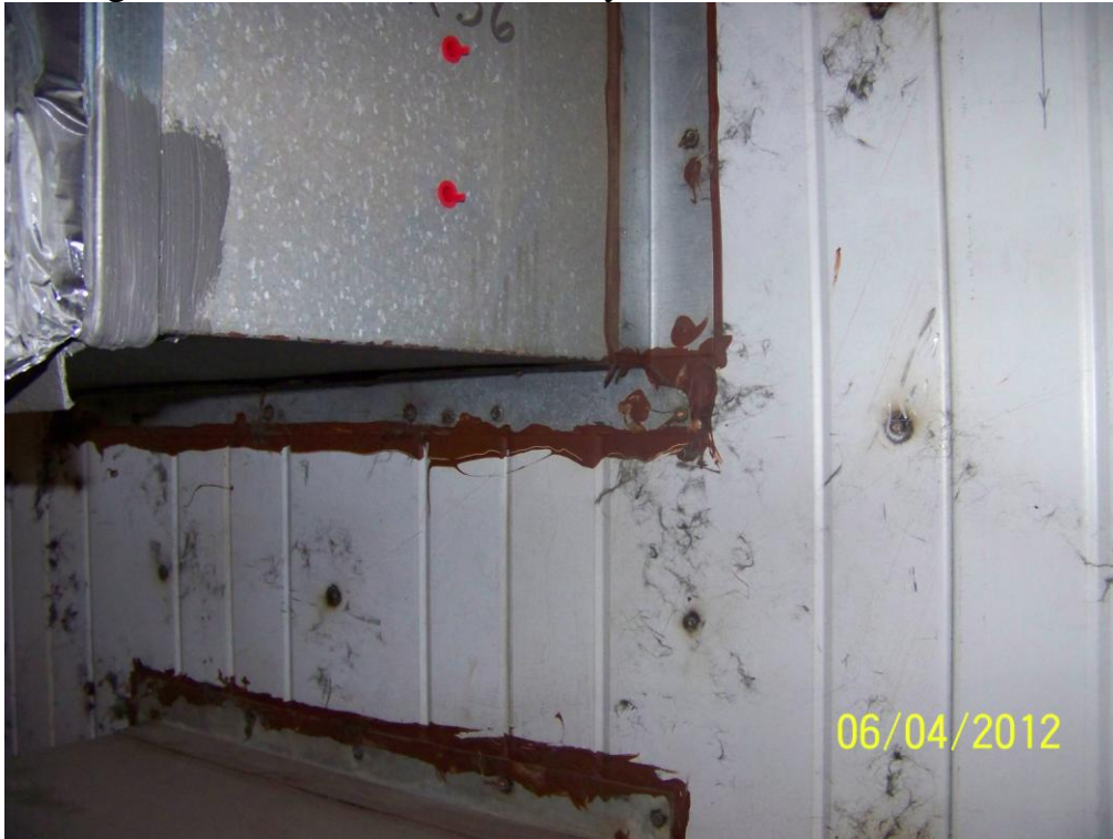
Homogeneous Material No. 5 – Putty, Red/Brown
