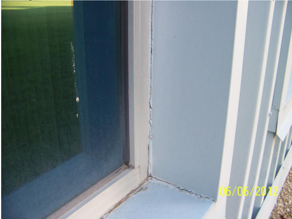
Homogeneous Material No. 35 – Exterior Window Caulk, Gray
