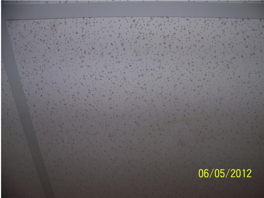
Homogeneous Material No. 23 – 2'x2' Ceiling Tile, White, Random Pin Holes and Gouges
