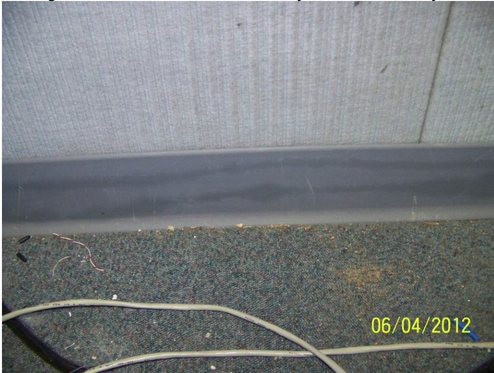
Homogeneous Material No. 15 – 4” Vinyl Cove Base, Gray
