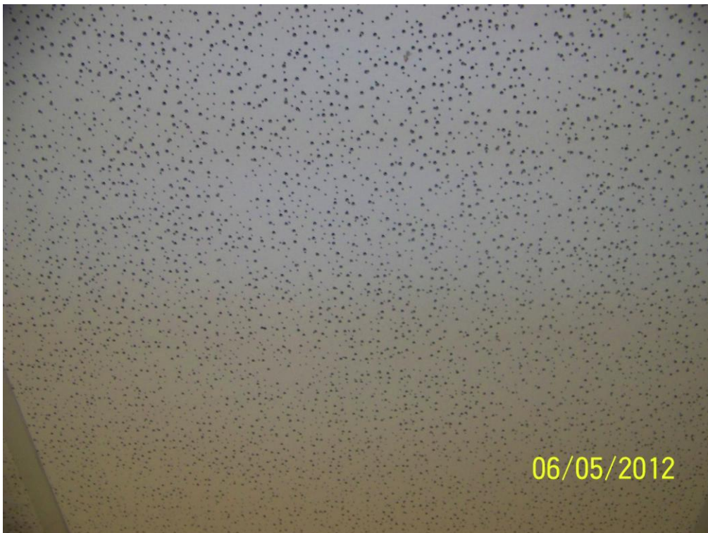
Homogeneous Material No. 28 – 2'x4' Ceiling Tile, White, Random Pin and Pen Holes
