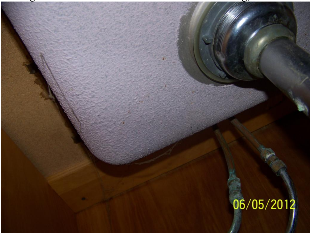
Homogeneous Material No. 24 – Under Sink Coating, White
