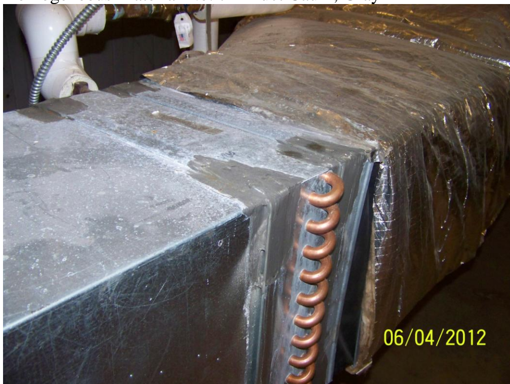
Homogeneous Material No. 7 – Duct Caulk, Gray
