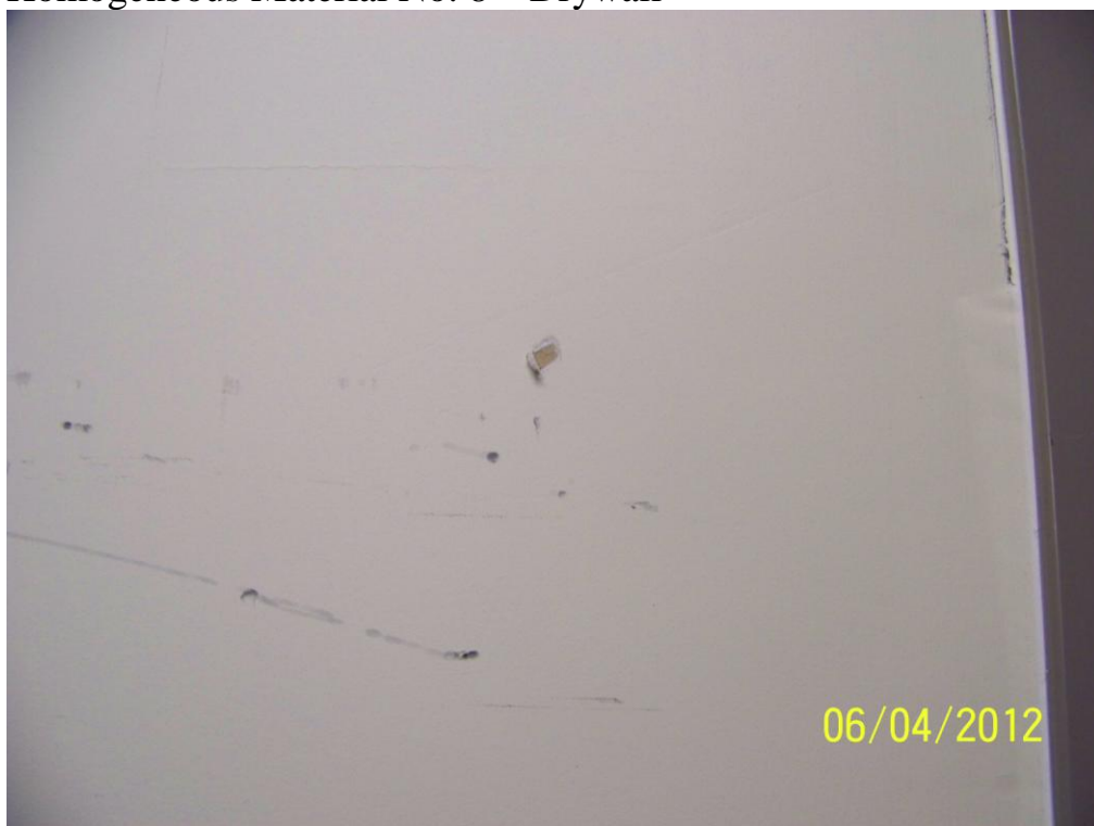
Homogeneous Material No. 8 – Drywall
