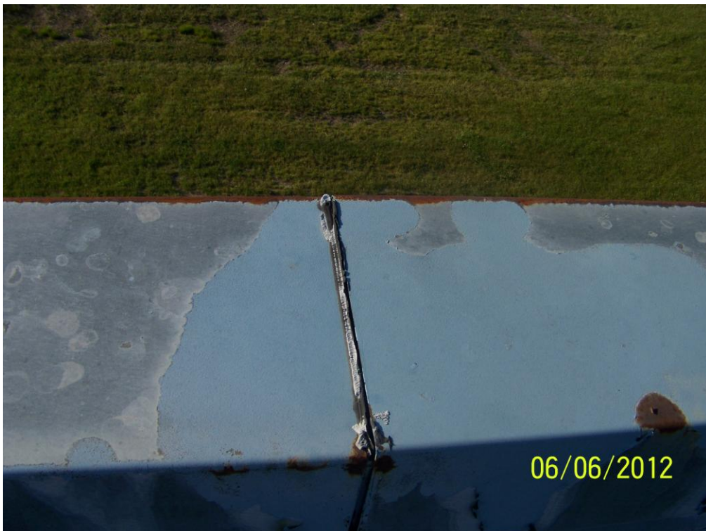
Homogeneous Material No. 34 – Exterior Roof Caulk, Black and White Mix
