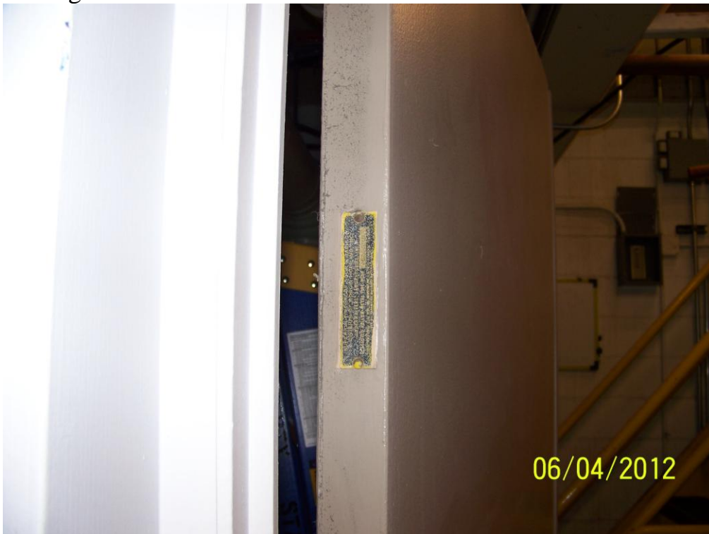
Homogeneous Material No. 2 – Fire Door
