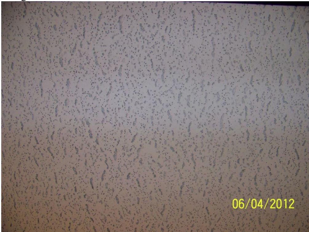
Homogeneous Material No. 12 – 2’x4’ Ceiling Tile, White, Lateral Gouges and Pin Holes
