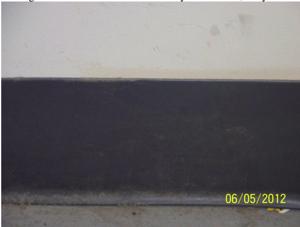
Homogeneous Material No. 25 – 6” Vinyl Cove Base, Gray
